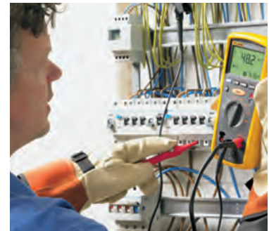
Insulation Test at a distribution Panel
